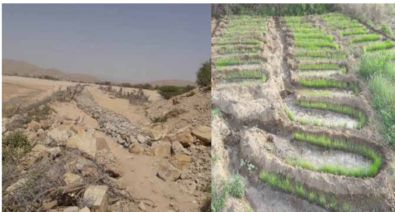
Photo: Flood diversion walls for farming fields in Habaas village in Zeylac district
